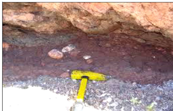
Fig.18. Fault gouge present in Chaibasa Noamundi Sub-Bain. Scale Hammer-31cm.
