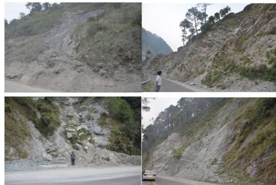
Fig. 5 Field photographs showing the various types of slope failures in the study area.
